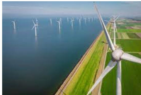
Windrad Off-/Onshore ca. 3,99 - 13,79 Cent / KWh
